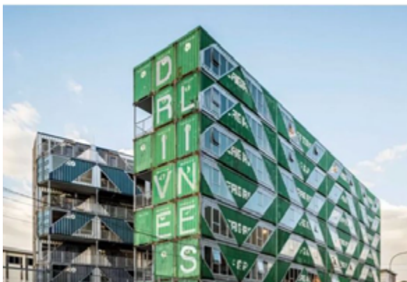
Жилищна сграда / Residential building
