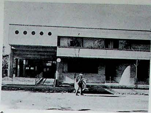
A project (scheme) for a school complex at Turgovishte. Location of the school in the civic centre, assuming cultural, educational and other functions, serving the population on integrative basis.
